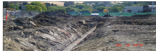
Storm water and sewer drain piping trench
